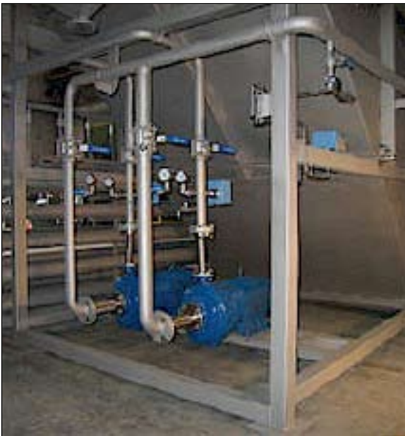
Figure 3: Installation of Shearforce Pumps installed in DAF application.
